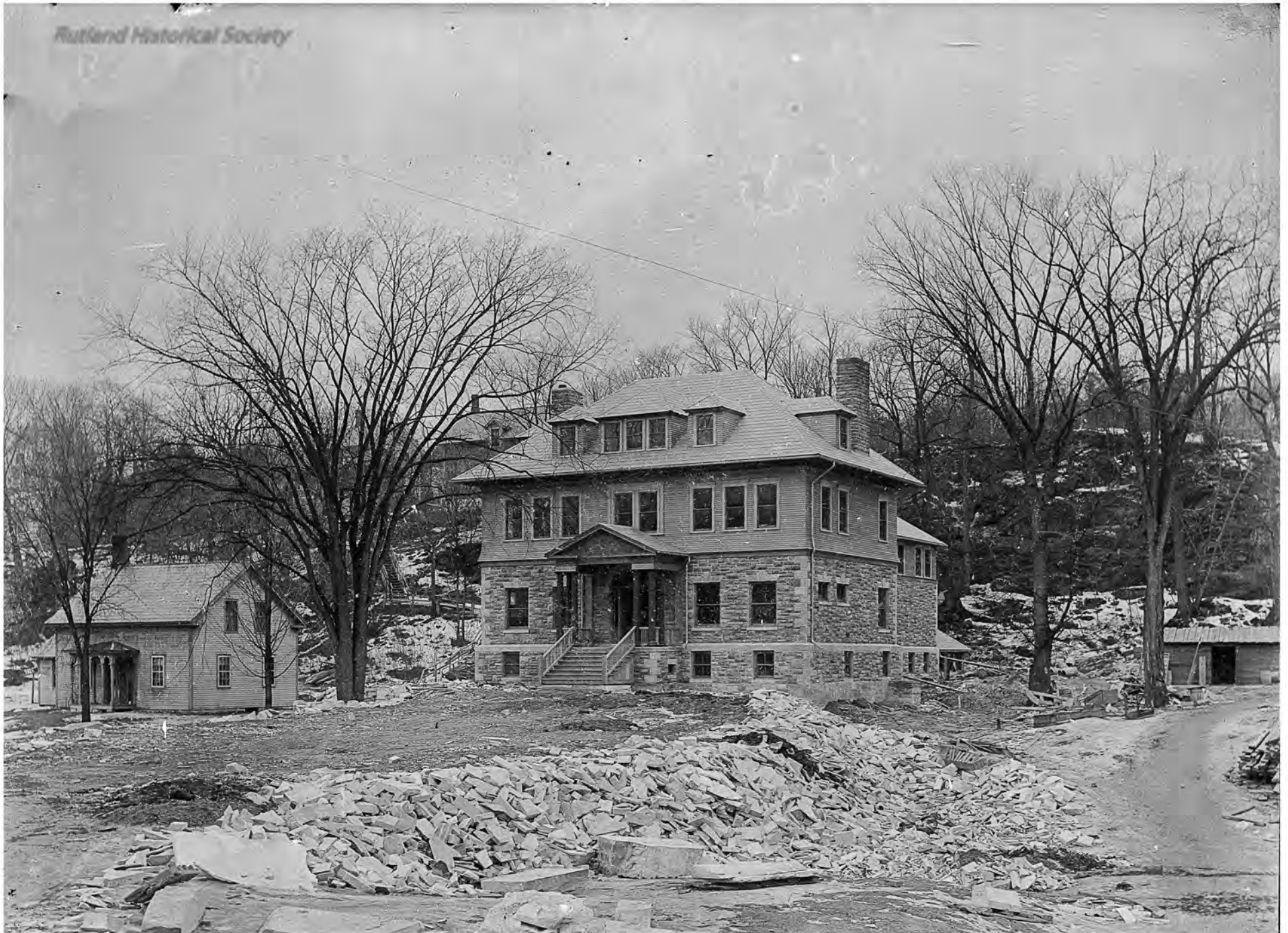
YMCA Building During Construction
